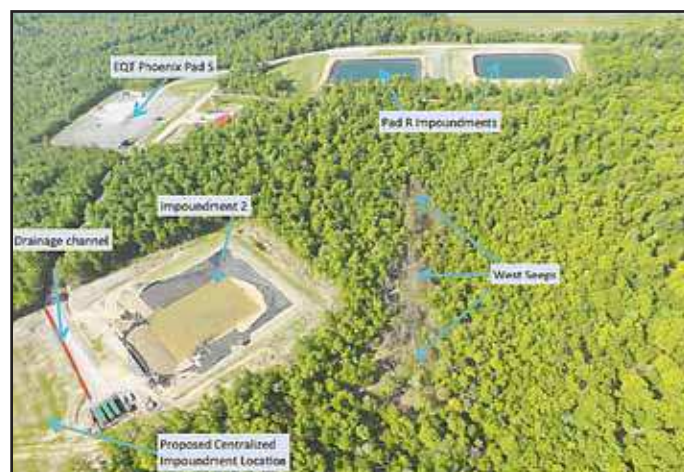
The Pennsylvania Department of Environmental Protection provided this aerial photograph, taken May 31, 2013, of the EQT Phoenix Pad S site.
